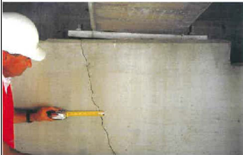
Diagonal Stress Crack in Under Beam
