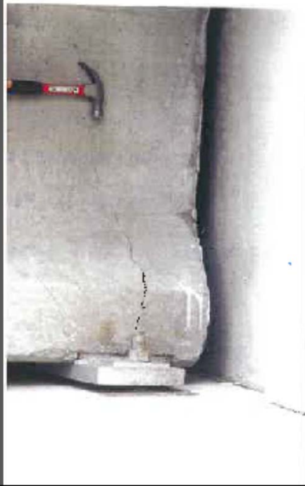
Vertical crack on beam web above bearing plate
